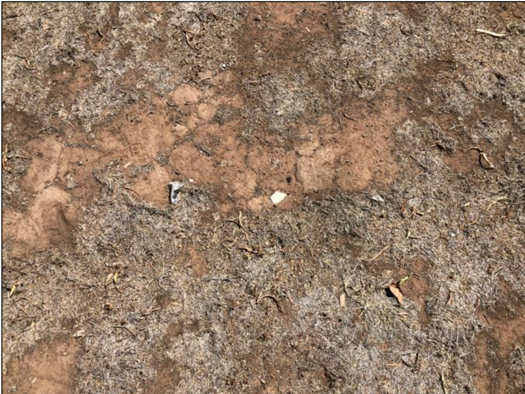
Figure 4.1: Photograph of Cement Sheet Fragments Observed on the Site Surface
